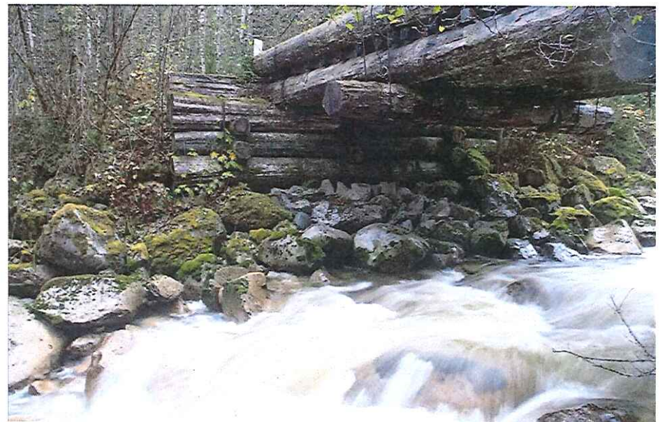
CK2232 Right Abutment
