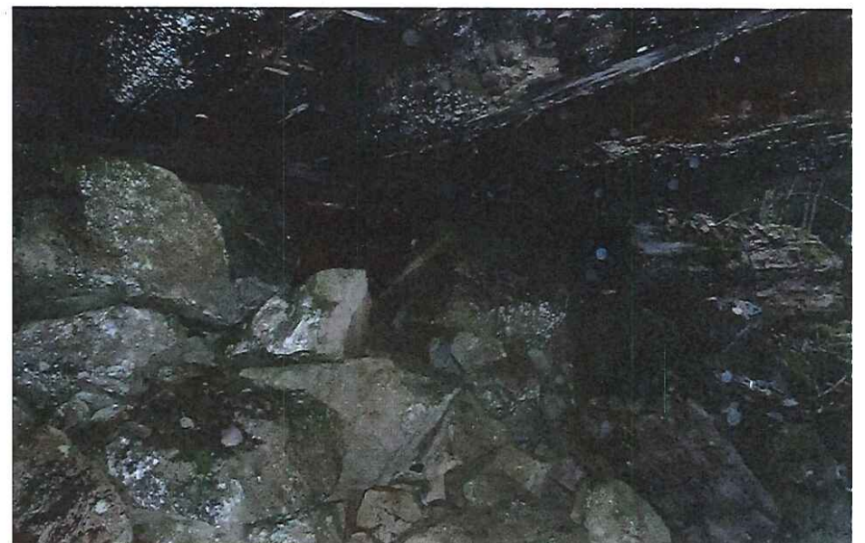
CK2232 Left Abutment
