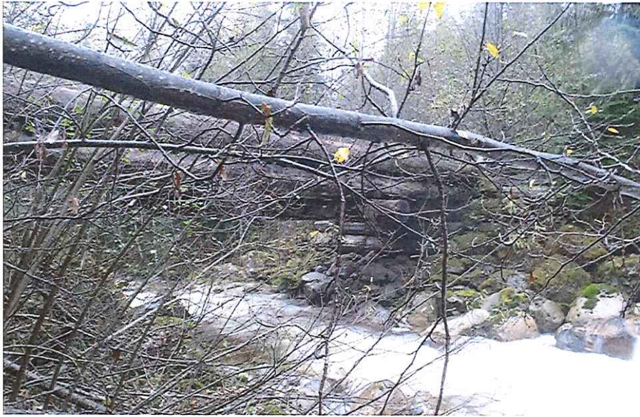
CK2232 Span 1 From Upstream
