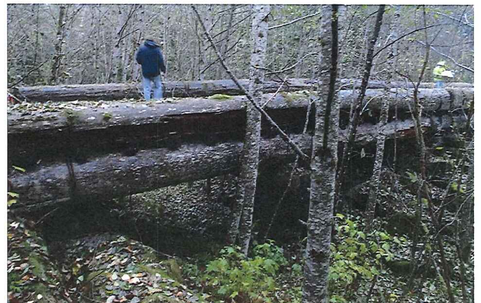
CK2232 Span 2 From Upstream
