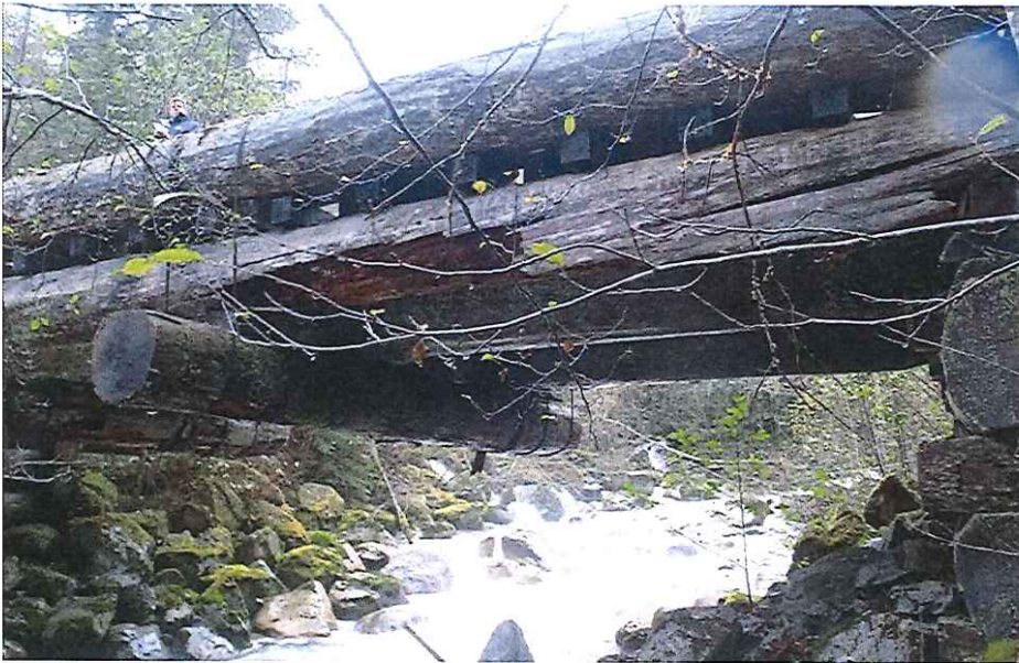
CK2232 Span 1 From Downstream
